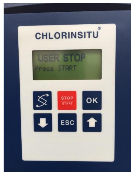
In this mode the water reservoir will be circulating without the production of chlorine. For this reason the reservoir will be free of chlorine in a short time. In this mode the brine pump can be set on 100% to flush the anode. Leave the unit for 15 minutes in this mode.
