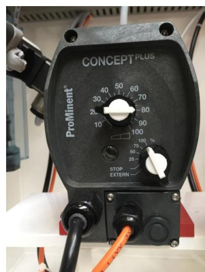
Put the brine pump on external position afterwards. Now the main power can be shut down . When the unit Will be in operation again, the STOP/START button can be pushed only and the unit will start production again.
